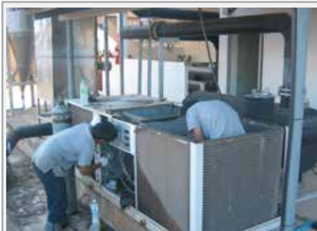
Repair/PM. Chiller, Heat pump
