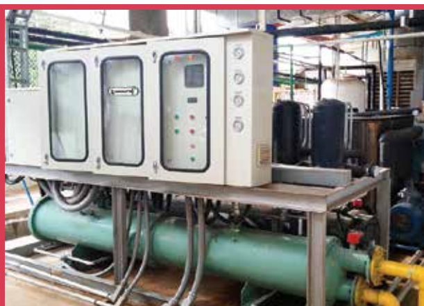
Water Cooled Chiller 140RT Water cooled chiller for process. Meadolc Asia.
